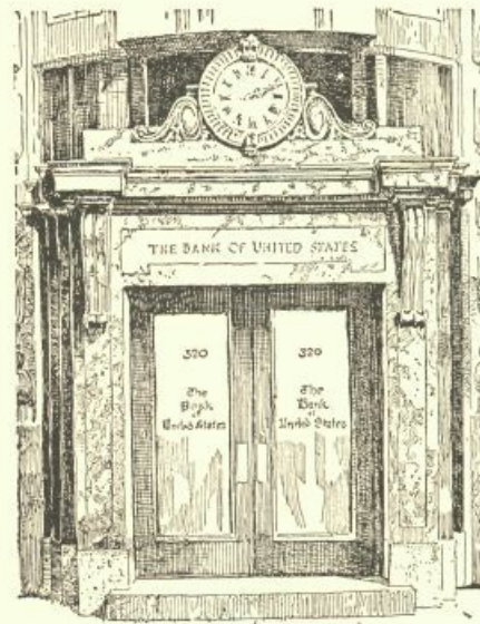
Entrance to Main Office
